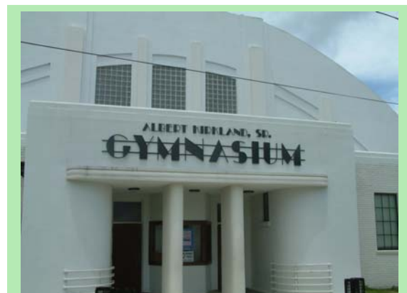
The renovations to the gymnasium portion of the Lake Wales Recreational and Cultural Centers are complete.
